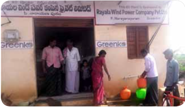
RO plant at Narayanapuram Village
