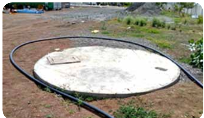
Rain water harvesting system at Wind Site
